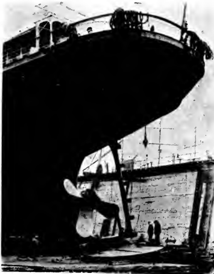
The steamer "Mimus" in dock receiving a new rudder.
